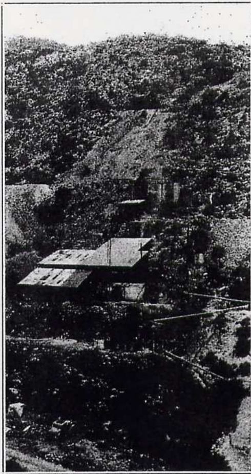
The 50-ton flotation mill recently completed by the La Bajada organization at the old Tip Top mine.
